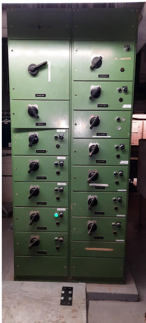
CD3 Motor control centres - wing C (front and rear)
