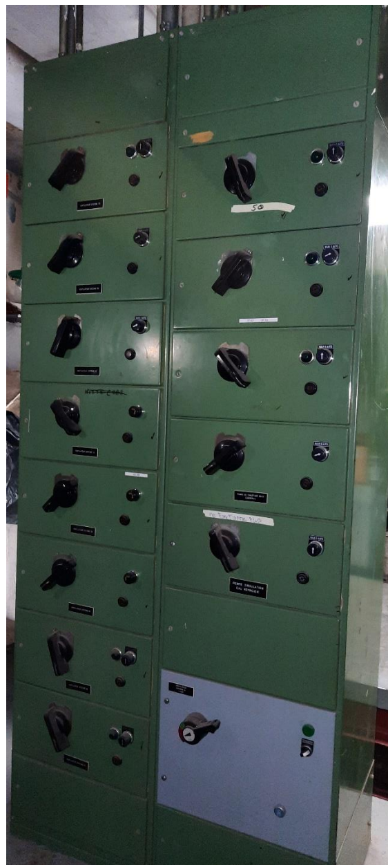
CD3 Motor control centres - wing C (front and rear)
