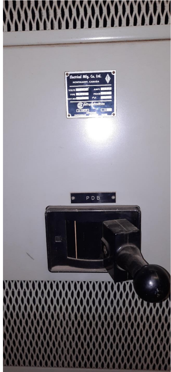
Distribution panel – Power Distribution Board (PDB)
