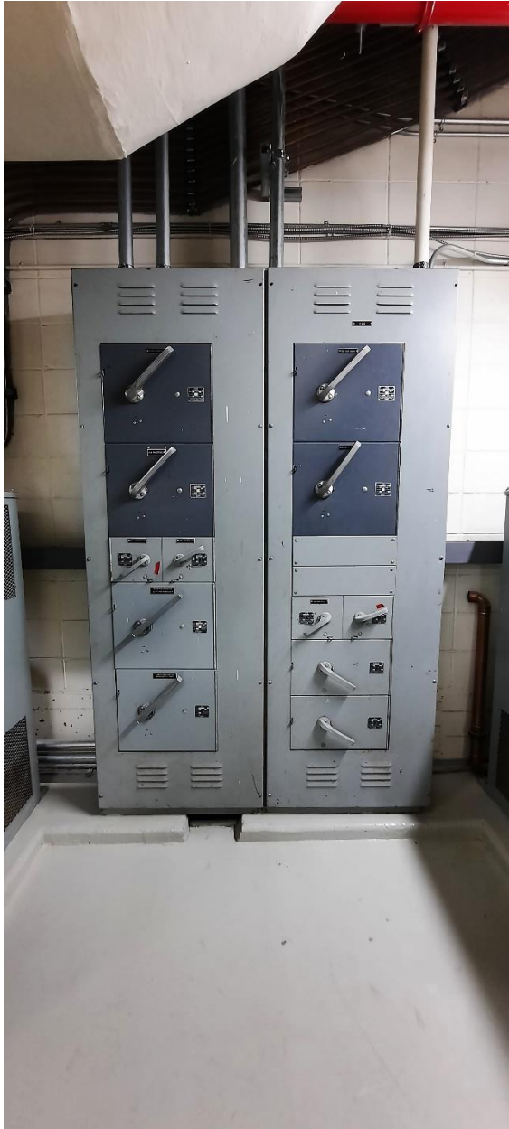
Distribution panel – Power Distribution Board (PDB)
