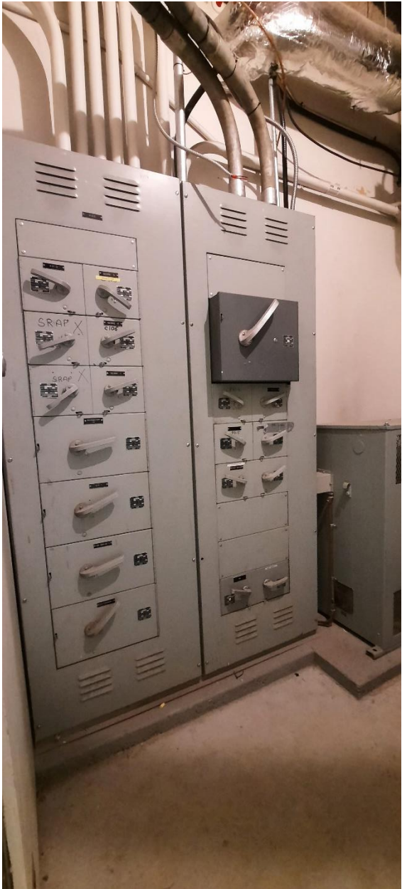
Distribution panel – Power Distribution Centre (PDC)
