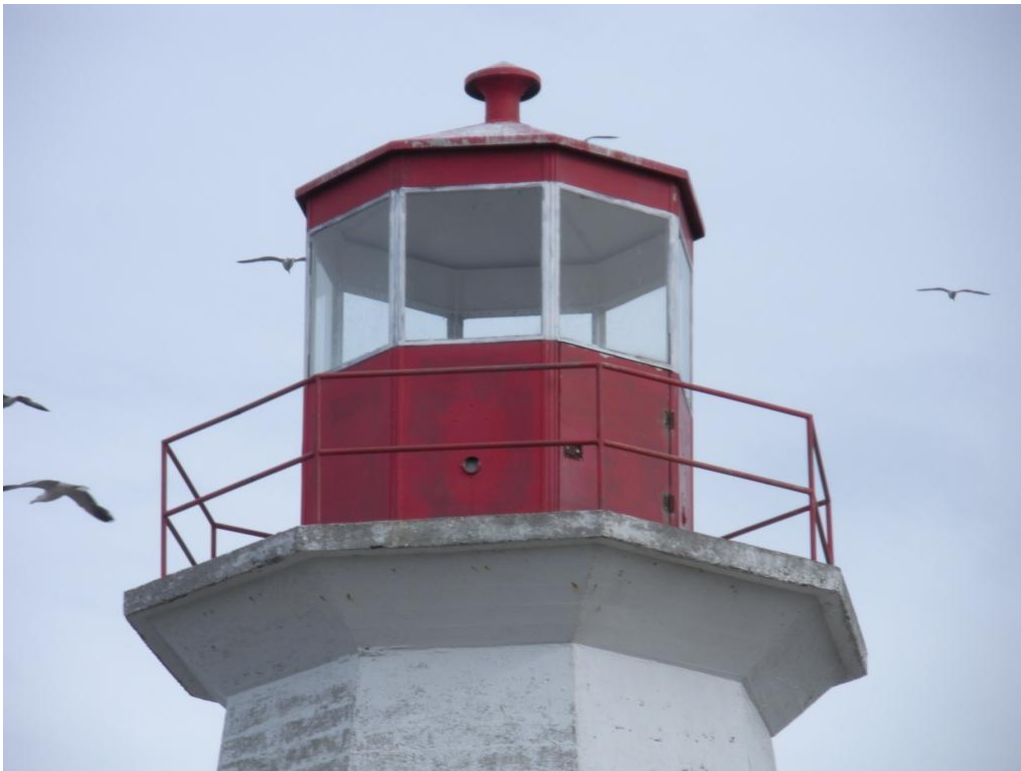
Photo 3 : View of the concrete balcony and steel dome
