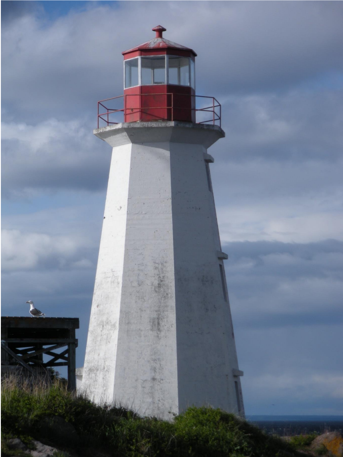
Photo 4 : Elevation view of lighthouse and windows
