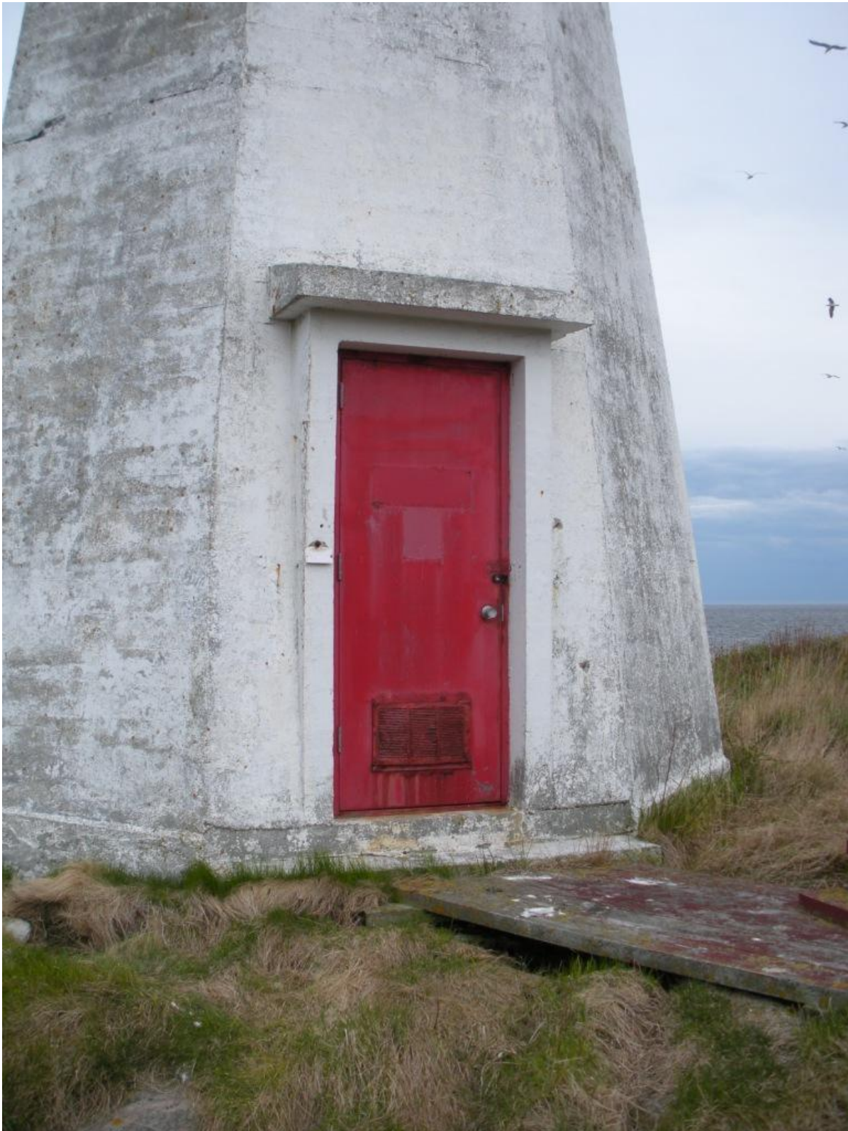
Photo 5 : View of front door to be scraped and repainted
