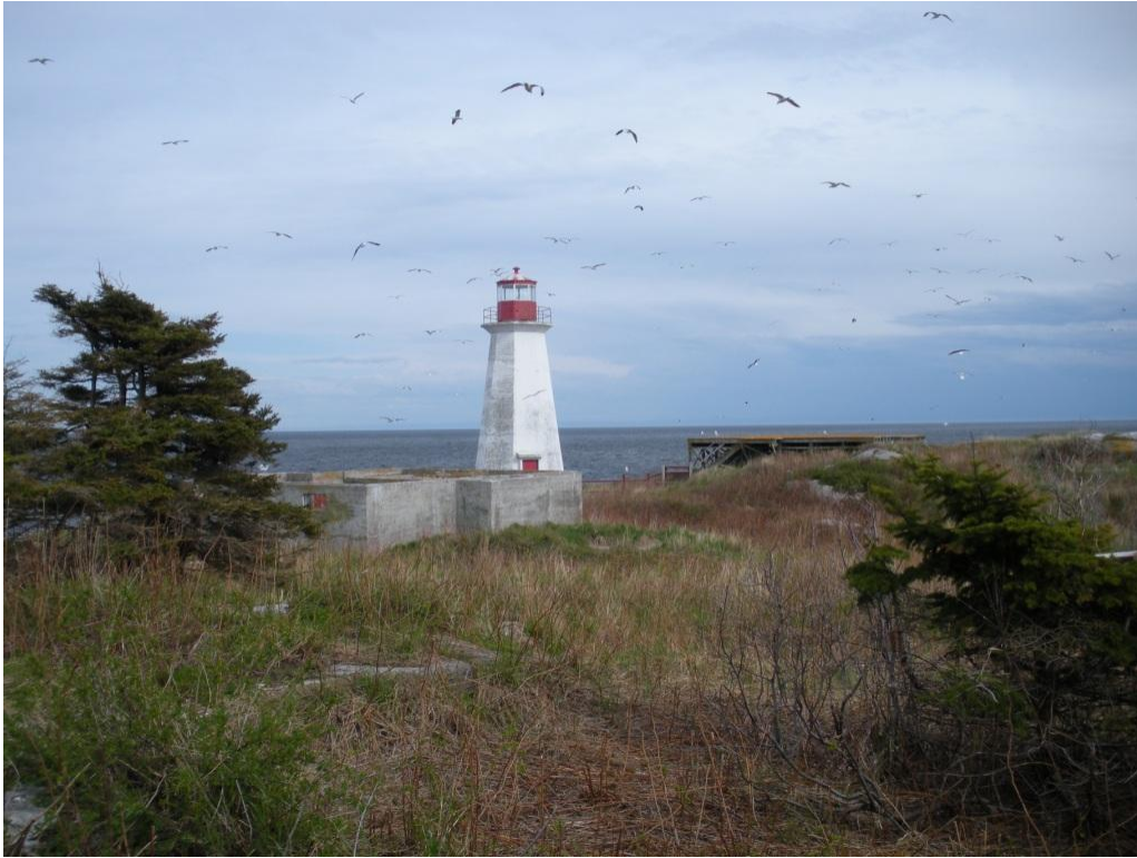
Photo 2 : General site view
