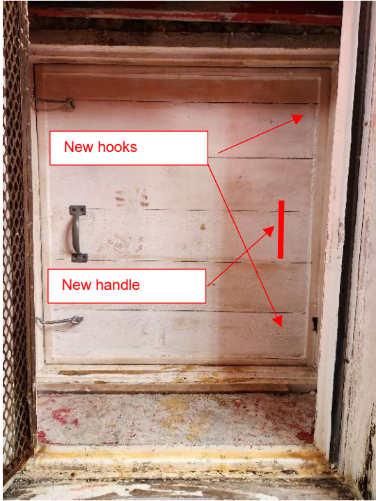
Figure 18: Exterior door for access to the gallery
