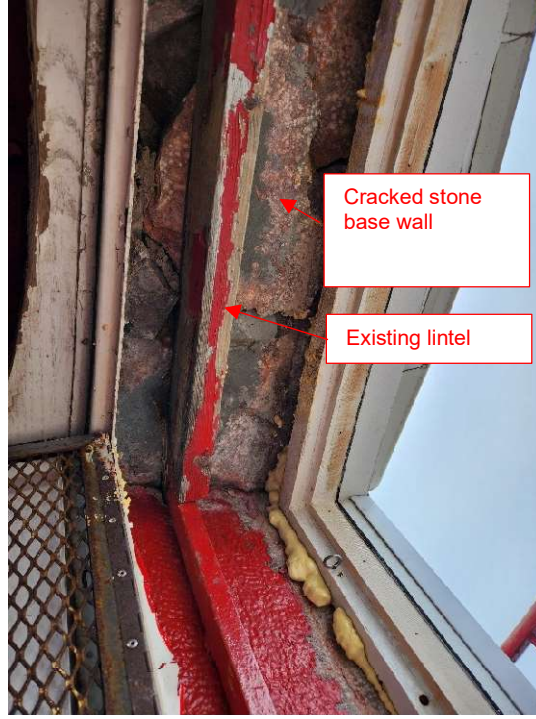
Figure 19: Gallery access door lintel
