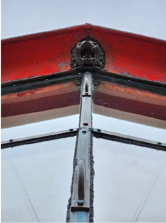
Figure 8: Glazing bead system that holds the glasses
