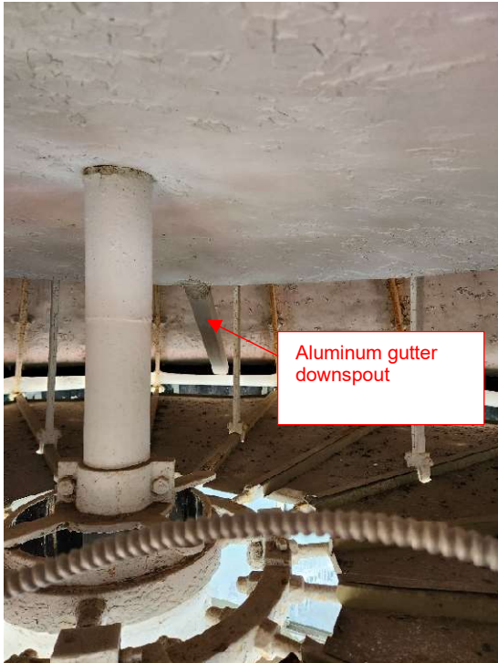
Figure 16: Location of the gutter downspout to be replaced.
