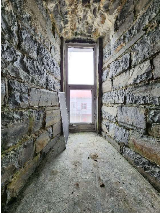
Figure 29: Typical tower window.
