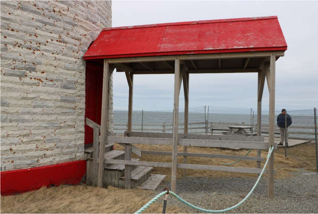
Figure 24: Wood pavilion to be dismantled and disposed.
