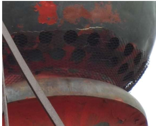
Figure 7 : Existing wire mesh held in place by
