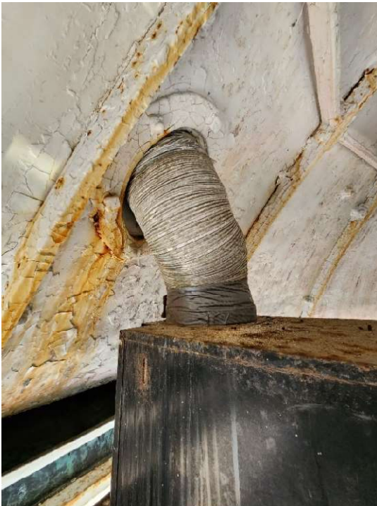
Figure 4 : Collar on the inner side
