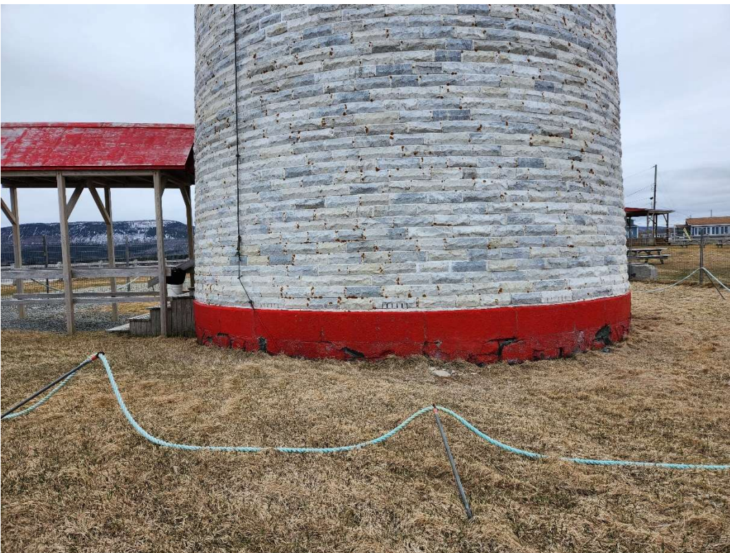
Figure 25 : Fence of rope and metal rods.
