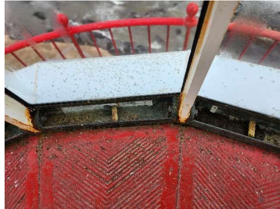
Figure 15: Aluminum Hatch and Hinge
