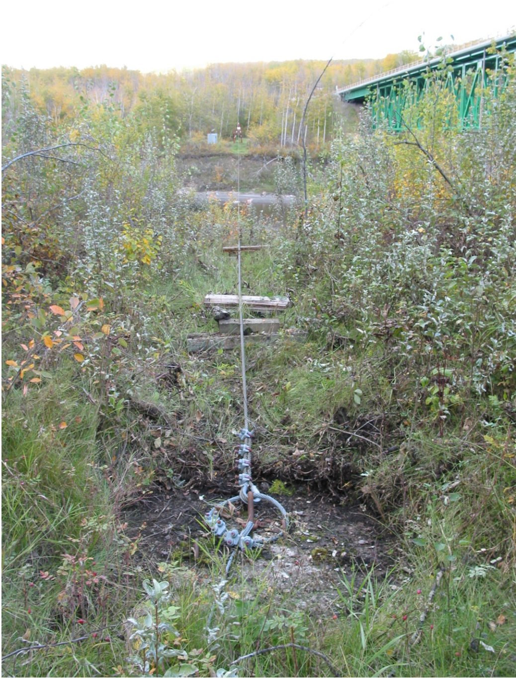
Figure 4: Infrastructure on Left Bank Far Side (Note: main center cable has been removed)
