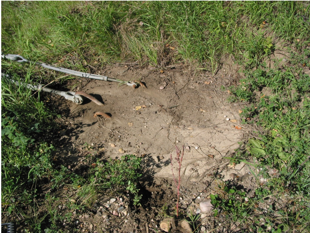
Figure 2: Concrete anchor on Right Bank Home Side
