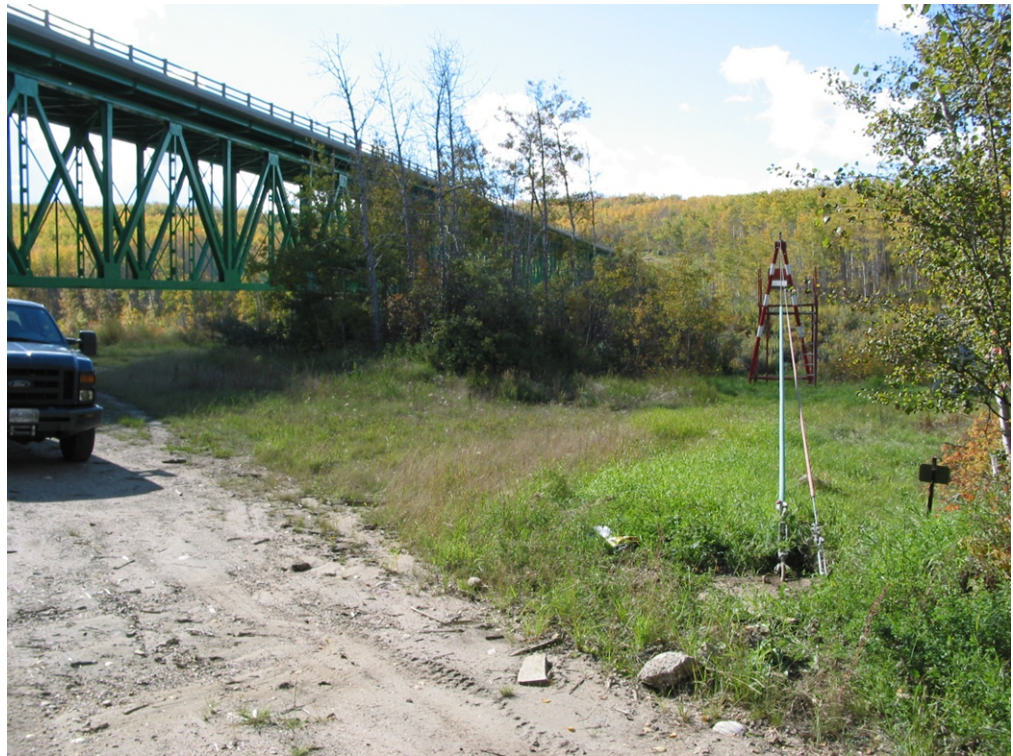
Figure 3: Infrastructure and surroundings on Right Bank Home Side
