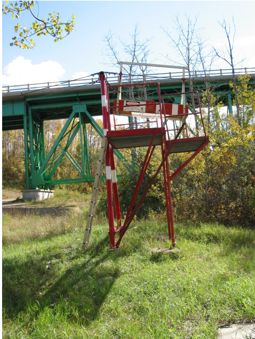
Figure 1: Existing tower on the Right Bank Home Side
