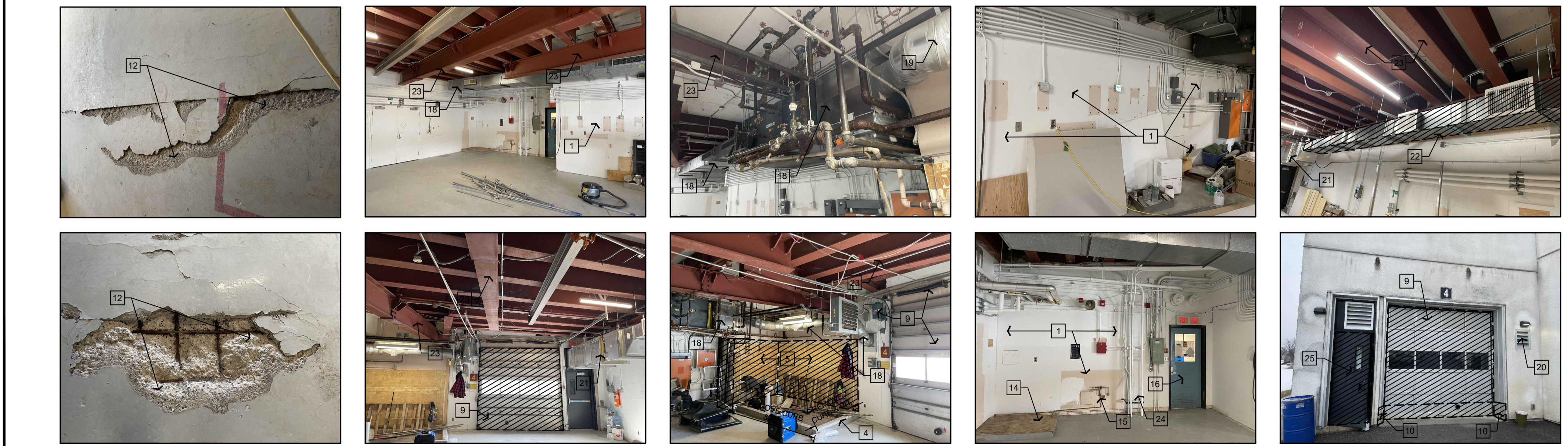
3 REFERENCE PHOTOS - EXISTING CONDITIONS SCALE = 1:50
