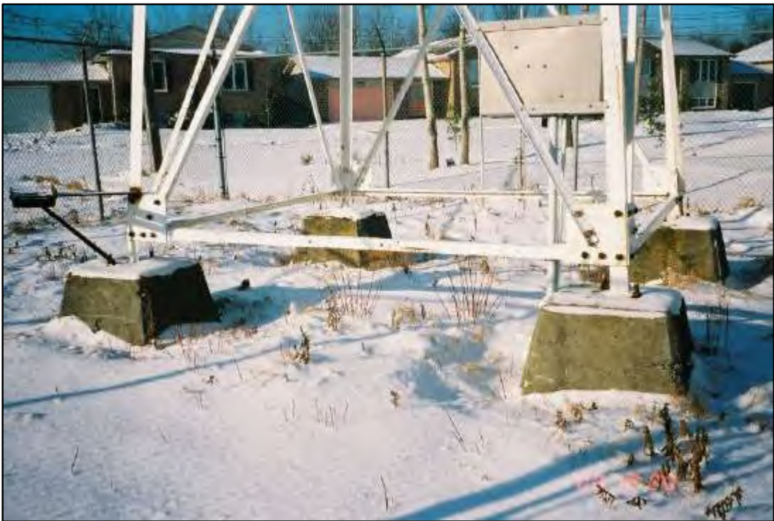
Photo 2. Base of Navigation Aid within fenced area.
