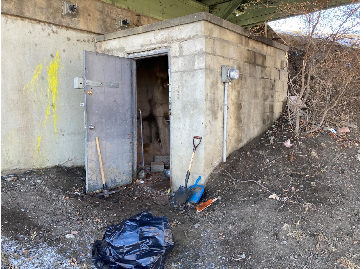
Figure 1: Existing structure - this will be removed by other Contractor
