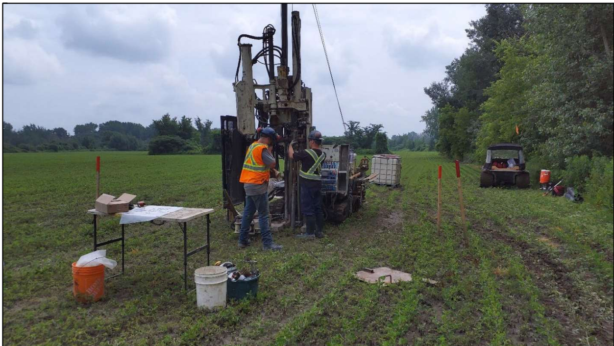
Figure 1 : Location of boreholes in line with the new RL (rear light) structure
