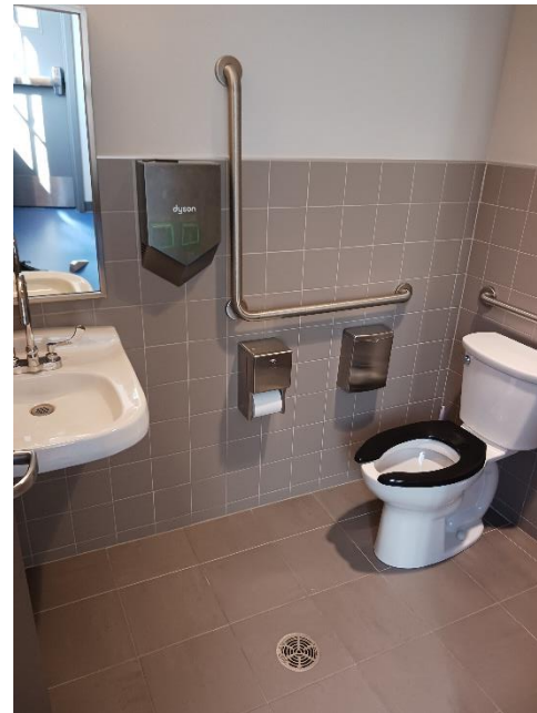
Lachine Canal Workshops: Restroom (room 208)
