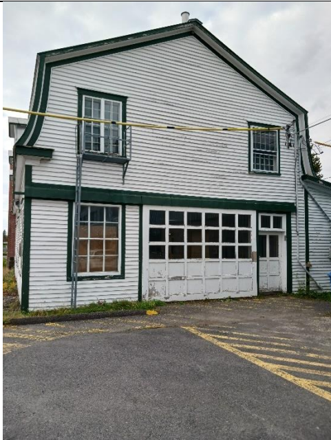
Chambly Canal Carpentry Workshops: Exterior
