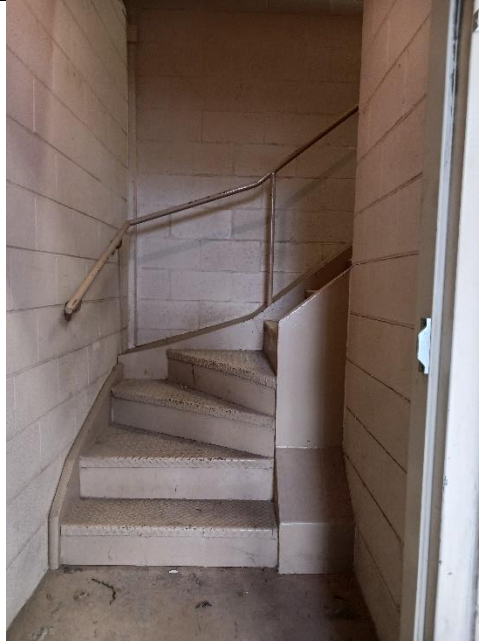
Chambly Canal Workshops: Stairs (ESC-D)
