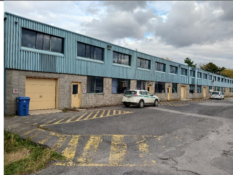
Chambly Canal Workshops: Exterior
