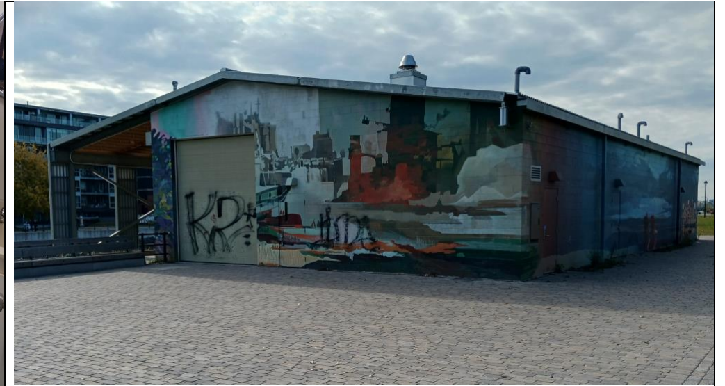
Hangar 1825 Restrooms: Exterior
