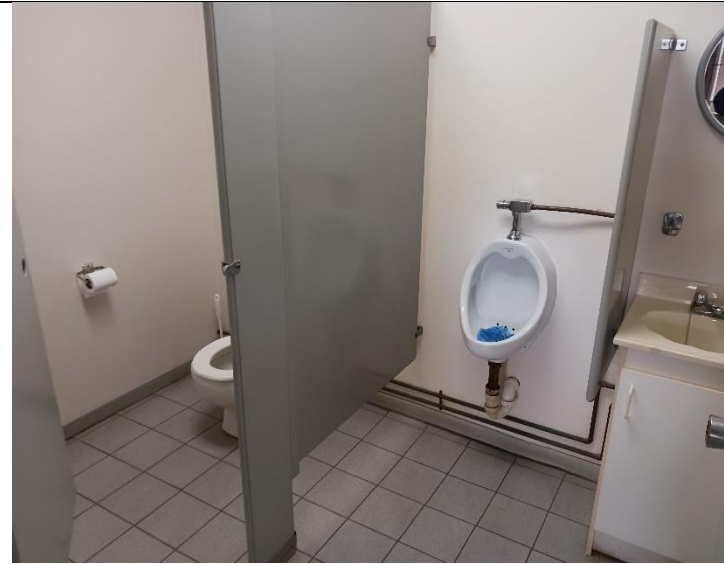
Chambly Canal Carpentry Workshops: Restroom
