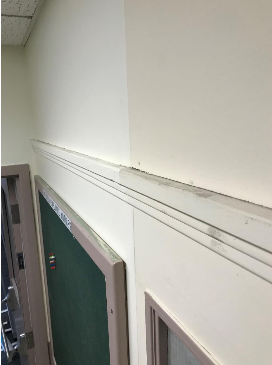
Photo 4: Transite panels observed on the wall between room 152 and 151 was confirmed to contain 1% Chrysotile asbestos (Historical Oakhill Sample ID 9698-U61 10A-C).
