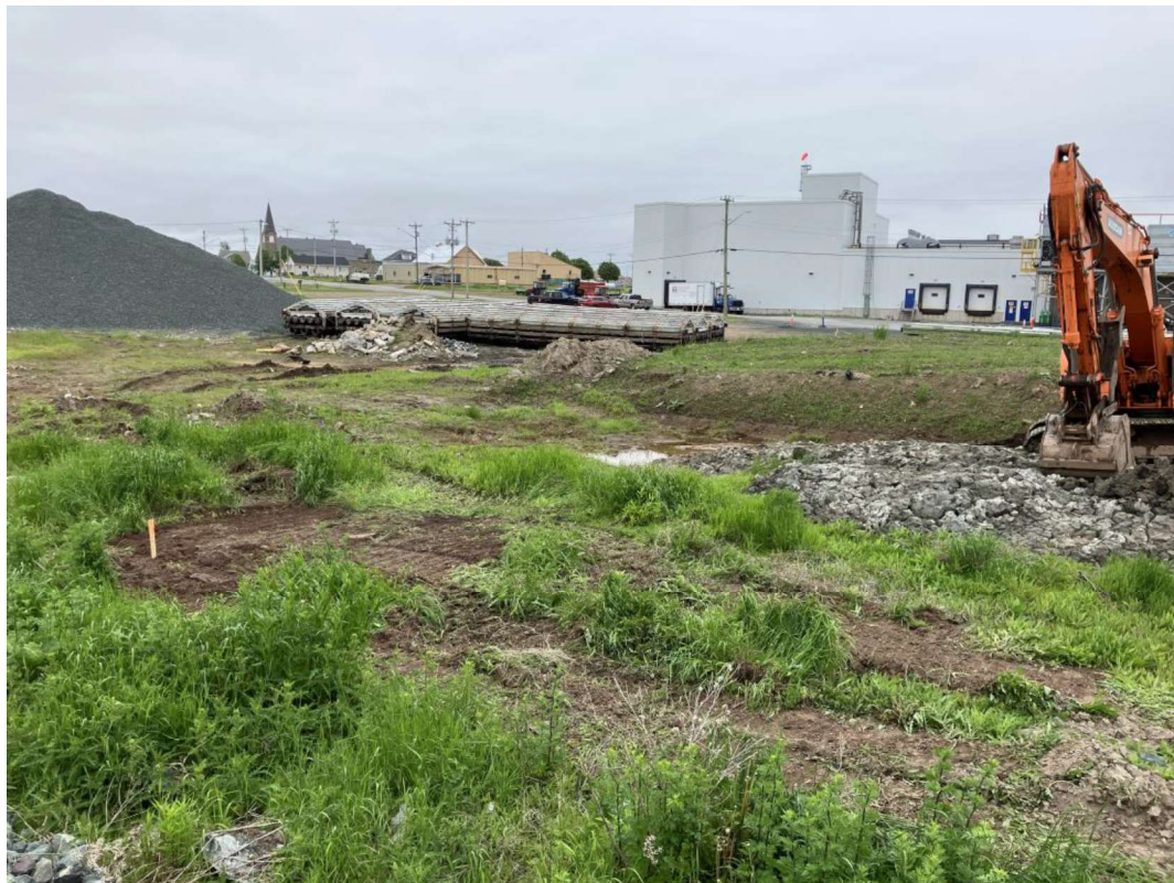
Photo 1: Containment Cell - General View, facing northeast
