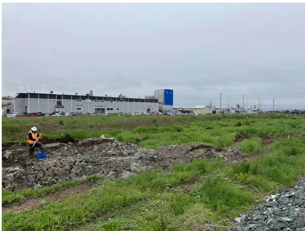
Photo 2: Containment Cell - General View, facing northwest
