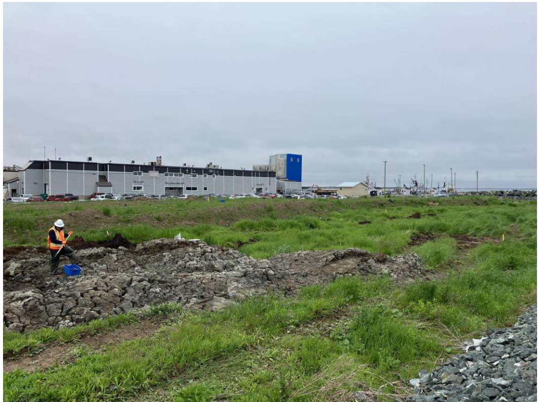
Photo 2: Containment Cell - General View, facing northwest
