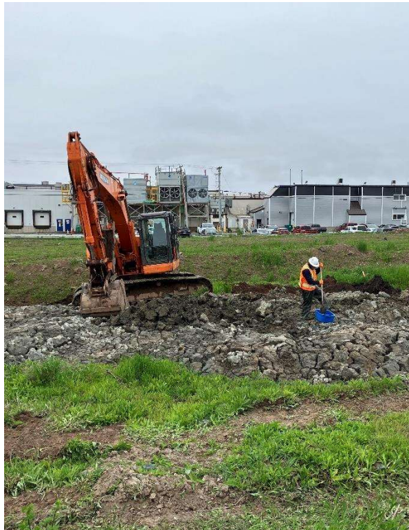
Photo 19: Sampling Location TP10
