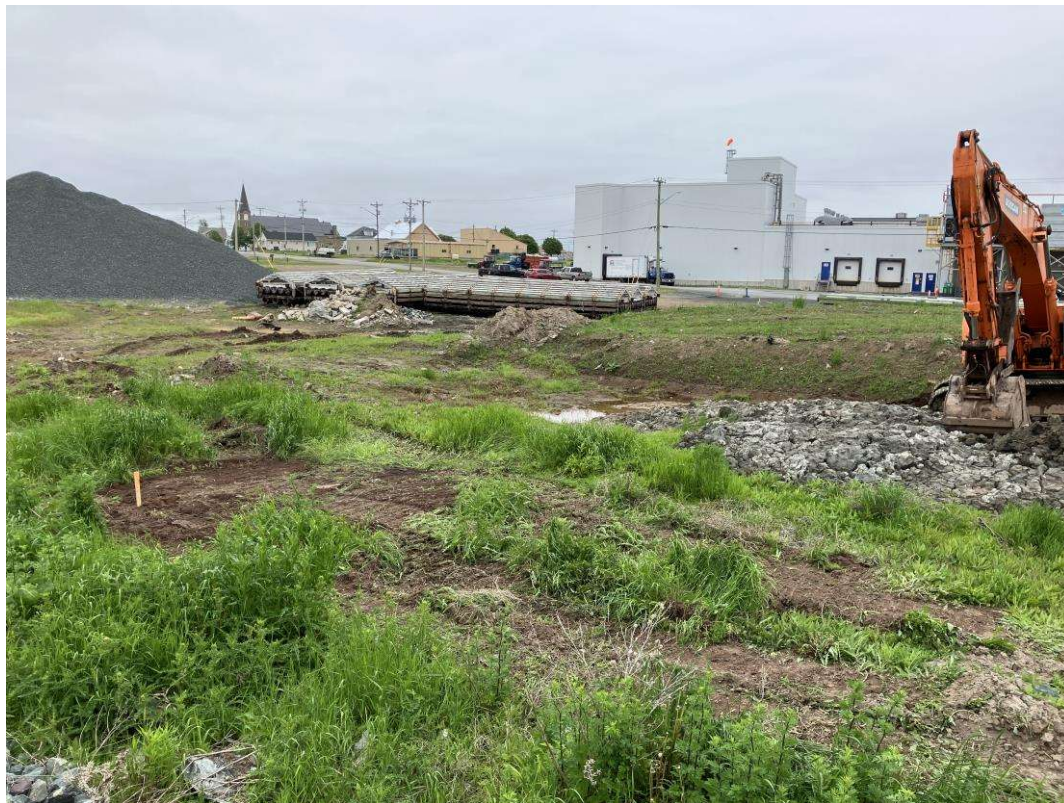
Photo 1: Containment Cell - General View, facing northeast
