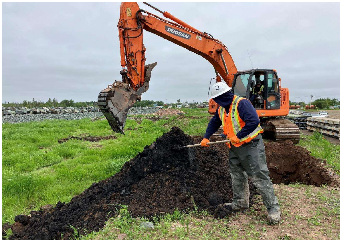
Photo 18: Sampling Location TP9
