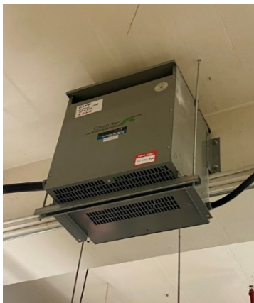
Figure 3-4 Examples of Installed Transformers Hanging from the Workshop Ceiling
