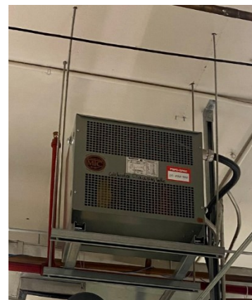
Figure 3-4 Examples of Installed Transformers Hanging from the Workshop Ceiling
