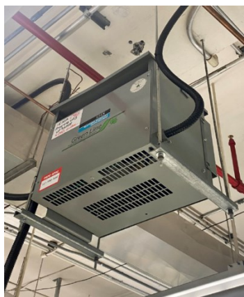
Figure 3-4 Examples of Installed Transformers Hanging from the Workshop Ceiling
