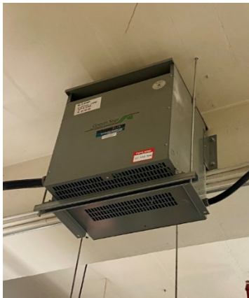
Figure 3-5 Examples of Installed Transformers Hanging from the Workshop Ceiling
