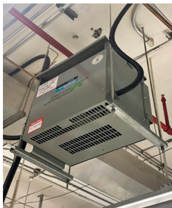
Figure 3-5 Examples of Installed Transformers Hanging from the Workshop Ceiling
