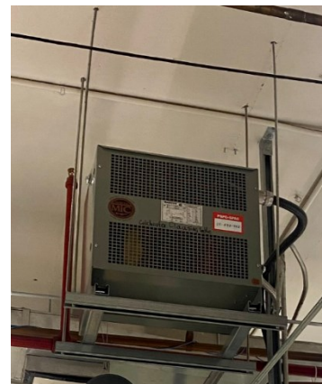
Figure 3-5 Examples of Installed Transformers Hanging from the Workshop Ceiling
