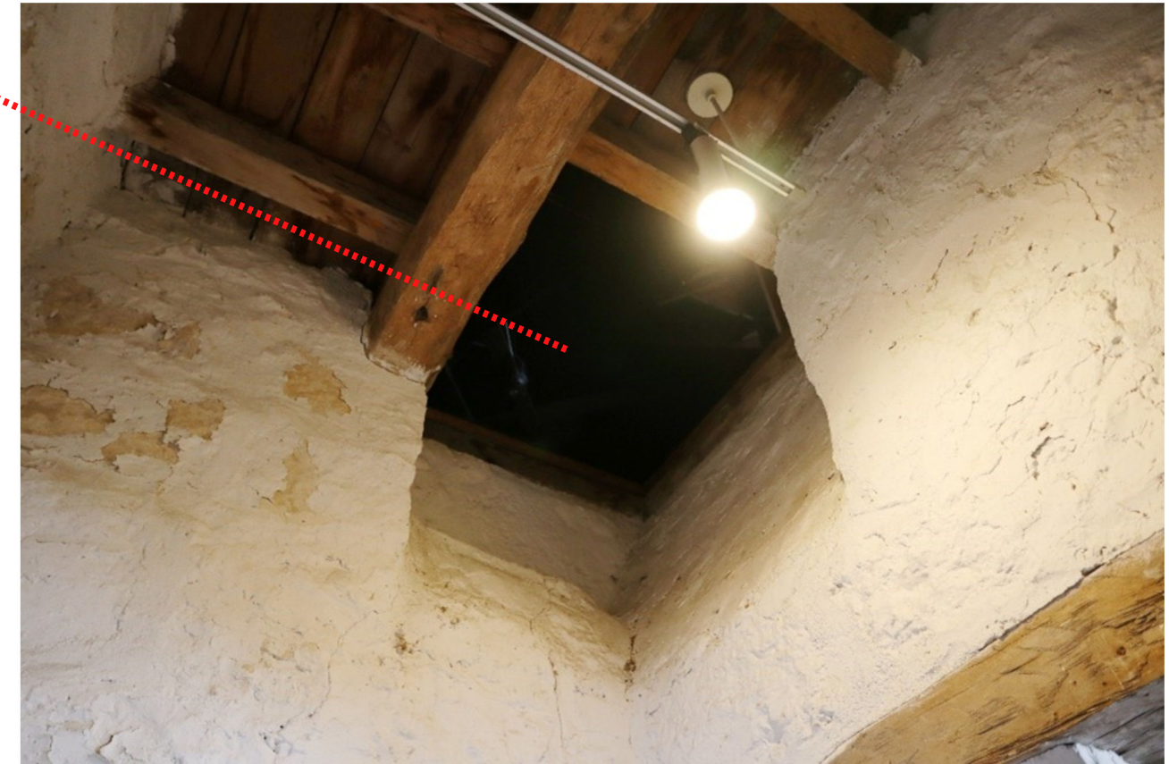
TRAP DOOR TO ATTIC, LOCATED IN VESTIBULE.
