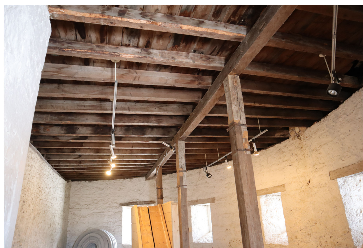
NORTH CEILING OVERVIEW
