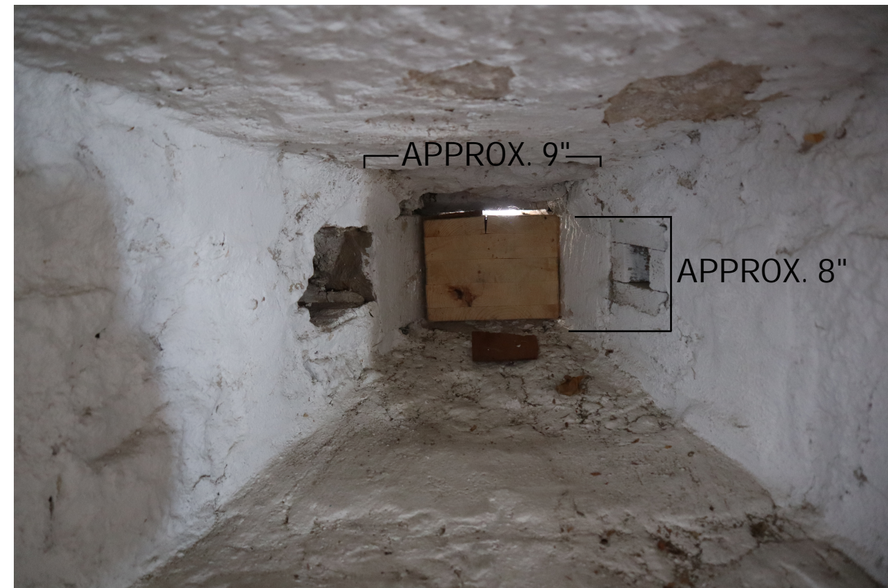
WINDOW #2, CLOSE UP
