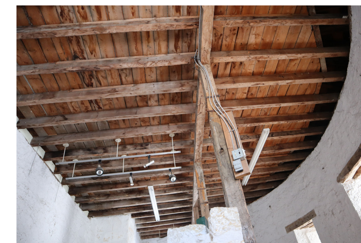
SOUTH CEILING OVERVIEW
