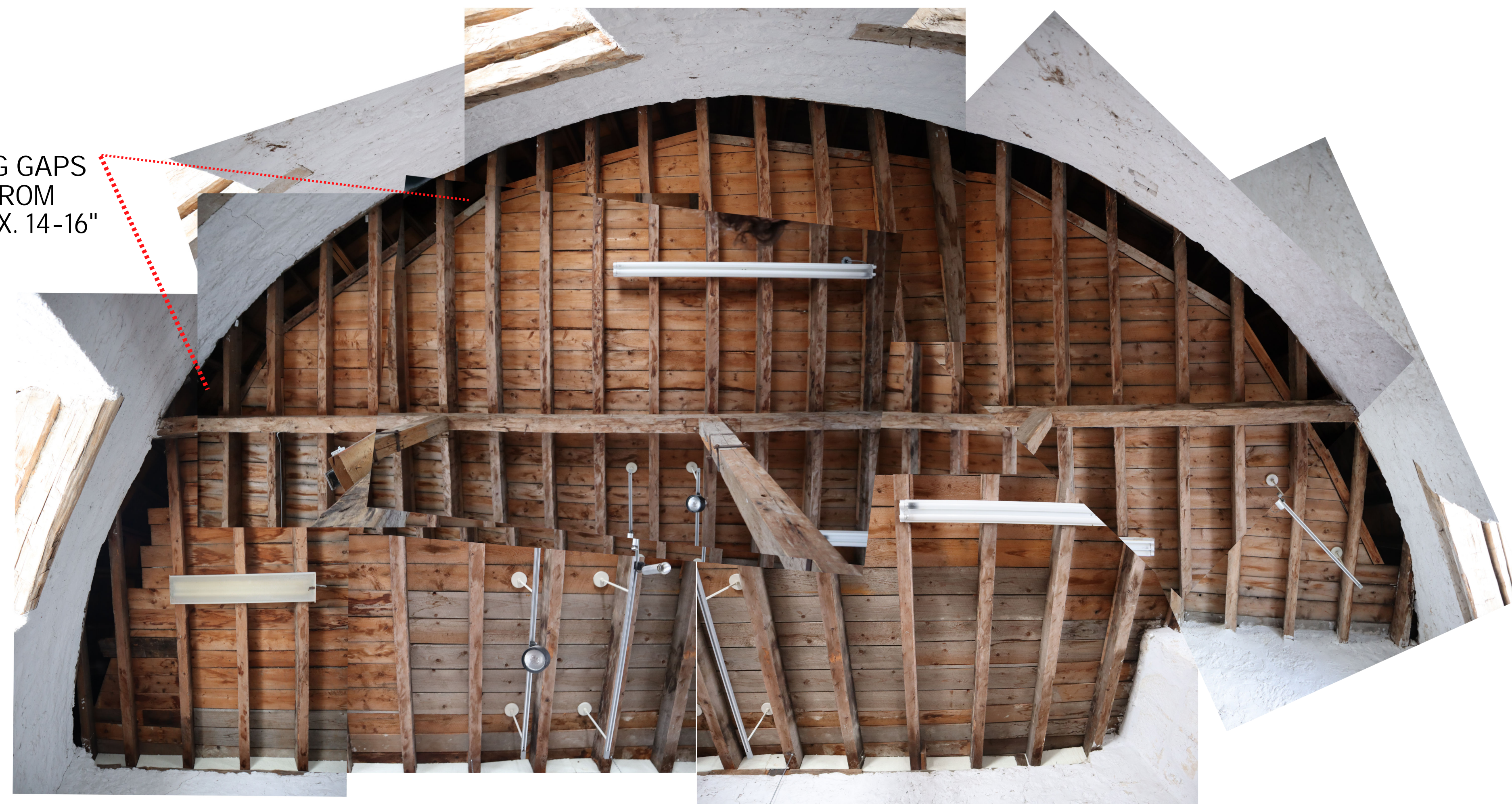
SOUTH CEILING FROM BELOW
