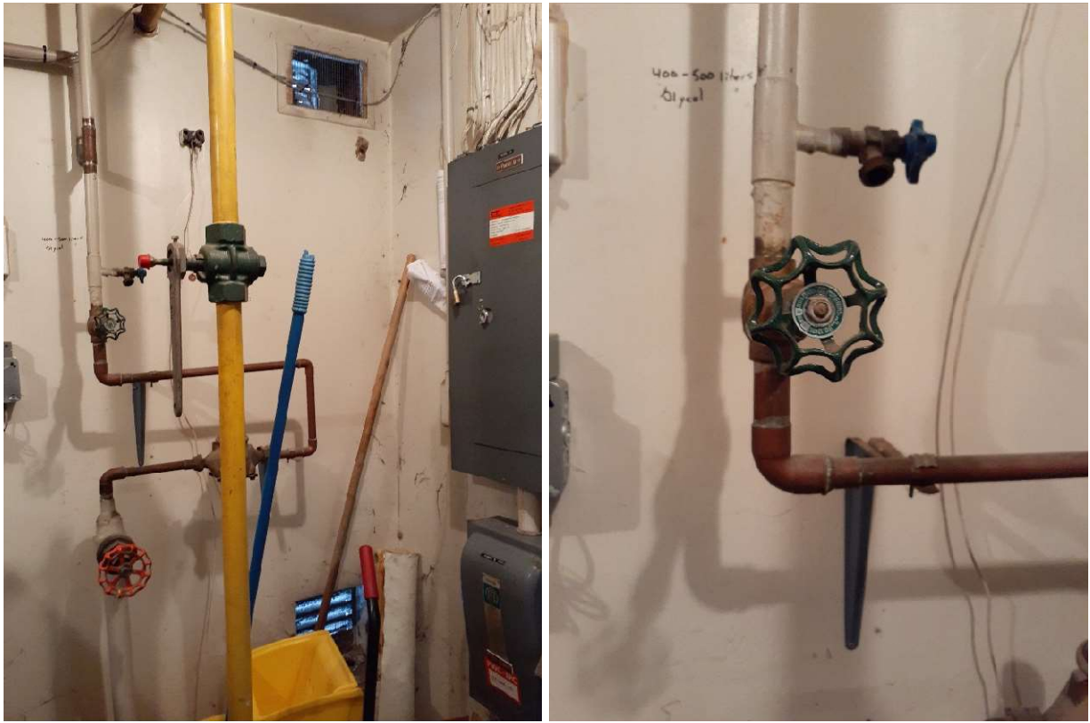
Figure 5: Representative photographs of the Mechanical Room in Building 141. Non-asbestos containing drywall joint compound located on the wall and ceiling [Sample ID: 141-AS-01A-C]. White paint on the wall [Sample ID: 141-LP-01; 1,900 ppm lead] confirmed to contain high levels of lead.
