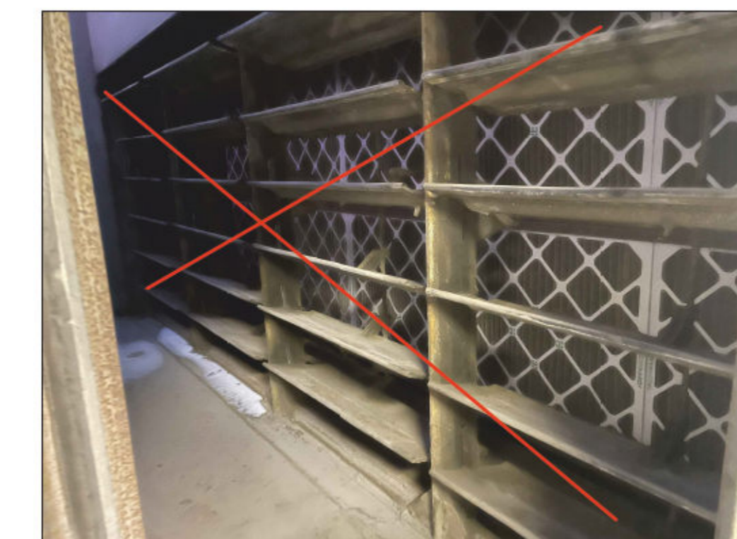
EXISTING DAMPER TO BE DEMOLISHED
