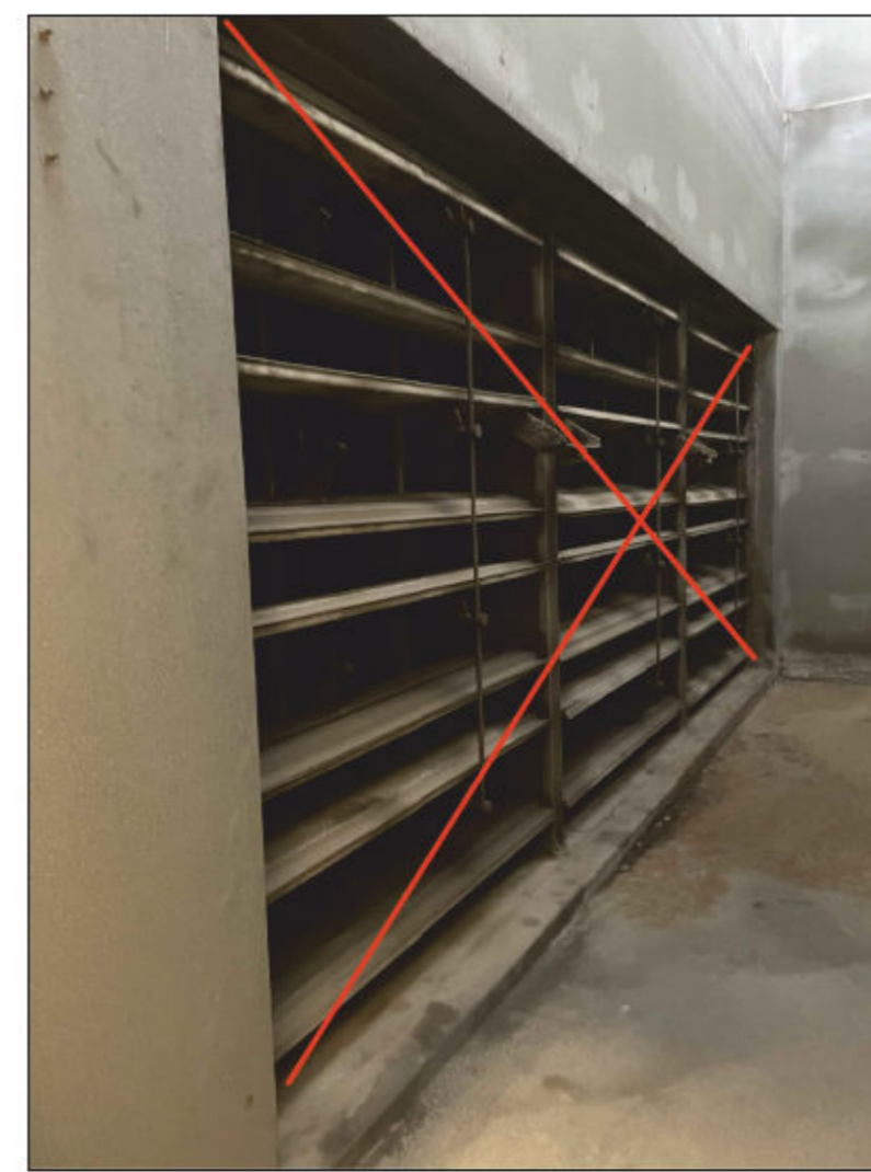
EXISTING DAMPER TO BE DEMOLISHED
