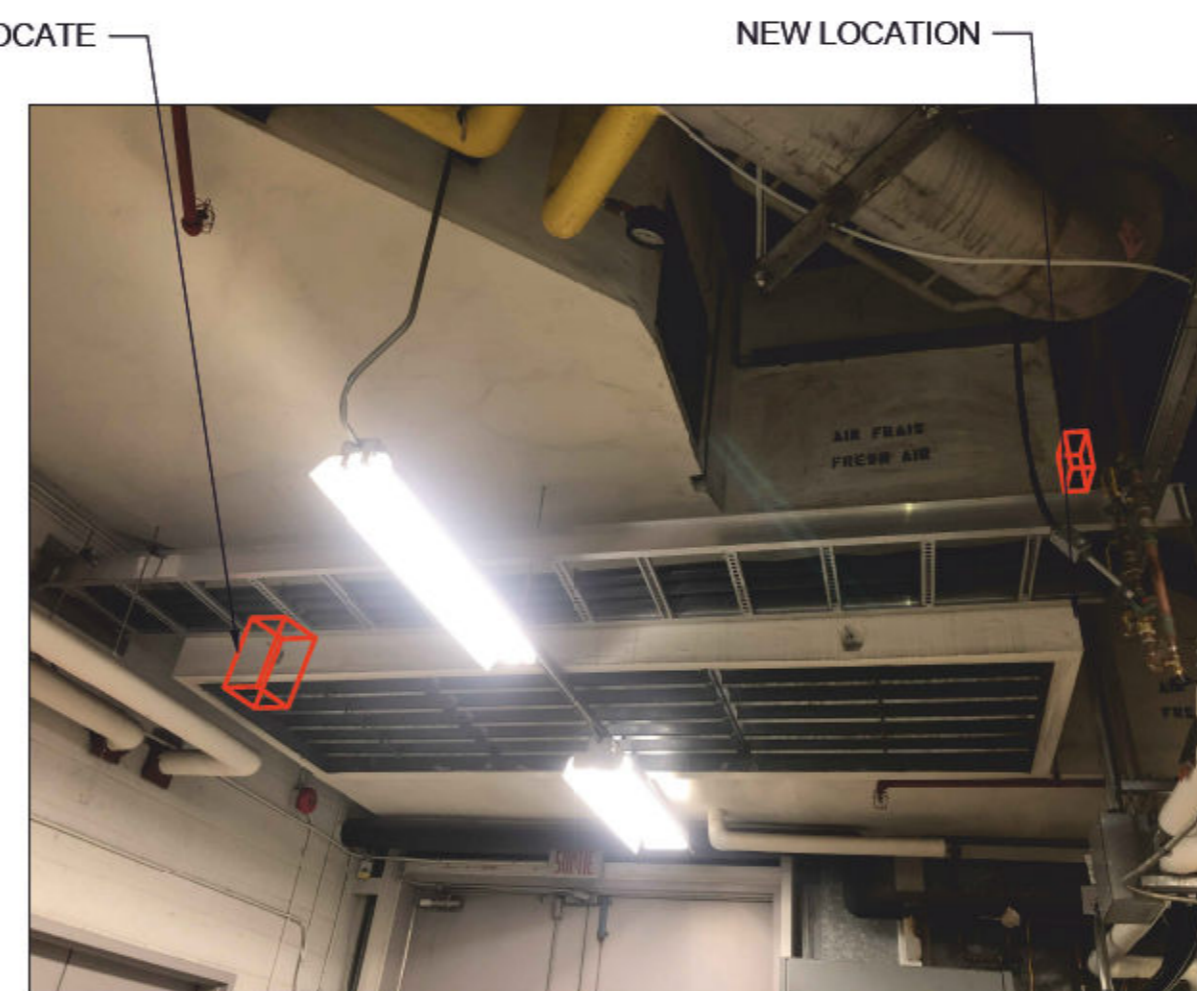
RELOCATION OF ACTUATORS LOCATION
