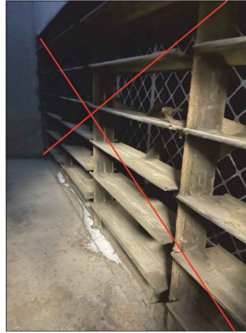
EXISTING DAMPER TO BE DEMOLISHED
