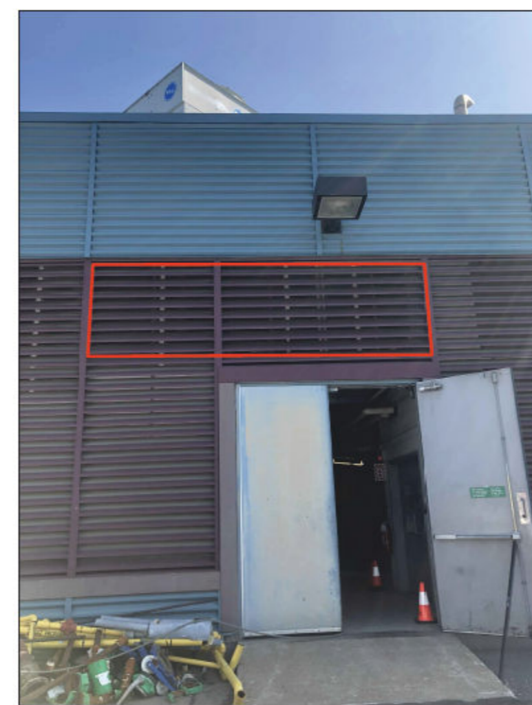
LOCATION OF MOTORIZED DAMPERS
