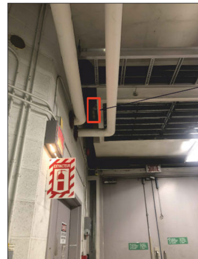
RELOCATION OF ACTUATORS LOCATION
