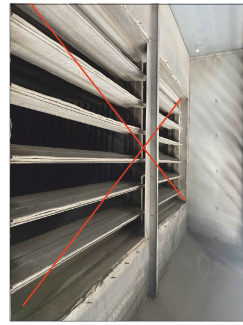
EXISTING DAMPER TO BE DEMOLISHED
