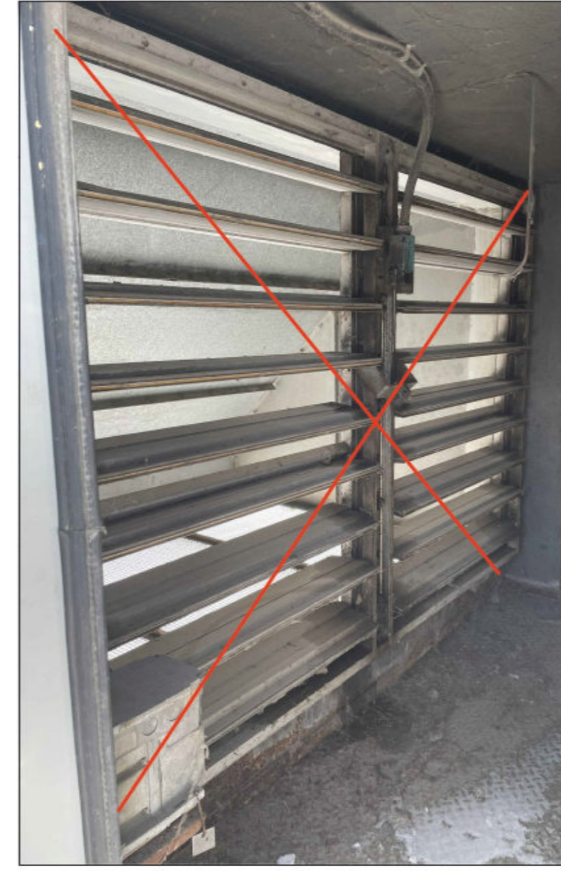
EXISTING DAMPER TO BE DEMOLISHED
