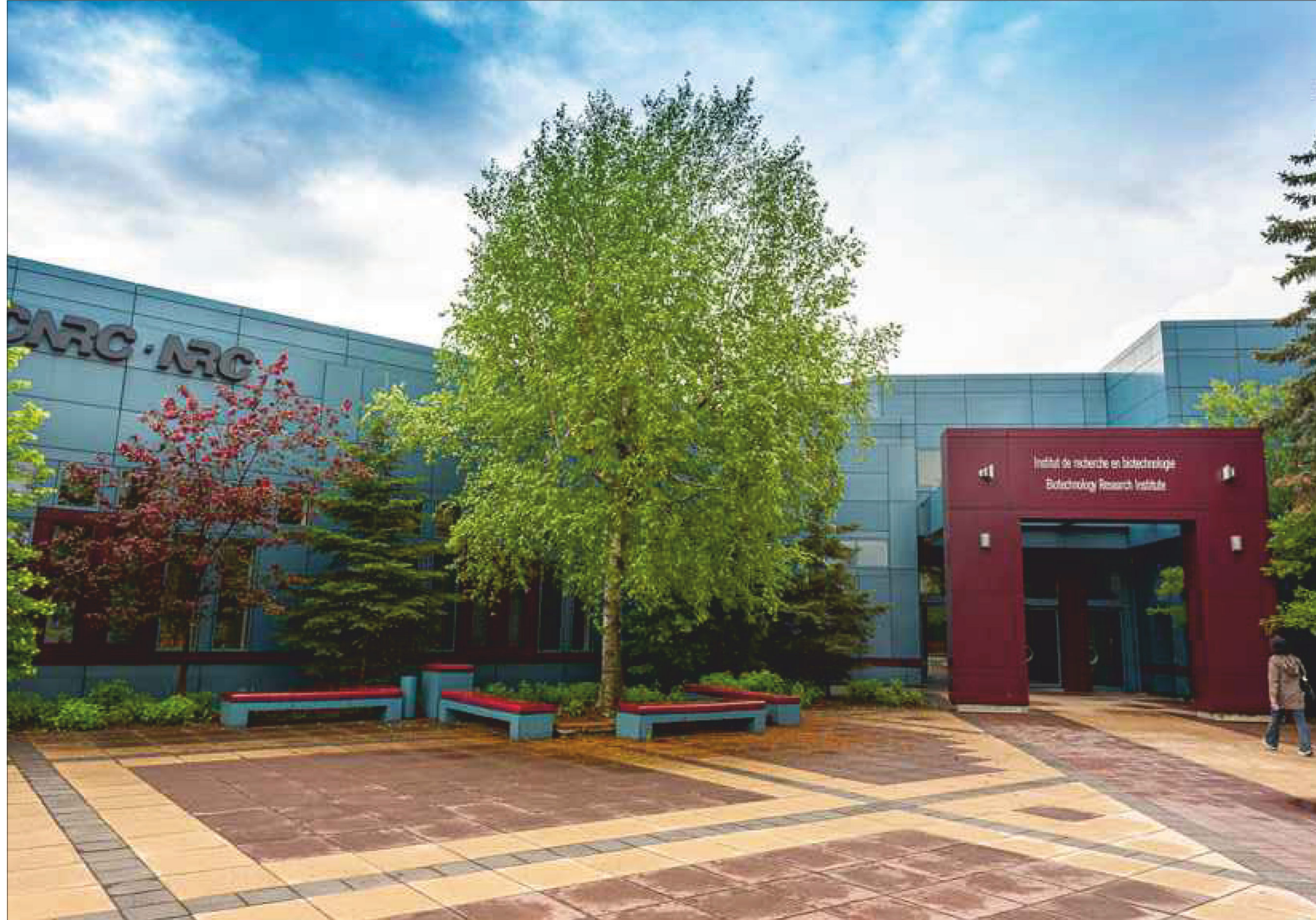
REPLACEMENT OF MOTORIZED DAMPERS 6100 Royalmount Avenue. Montreal, QC H4P 2R2, Canada
