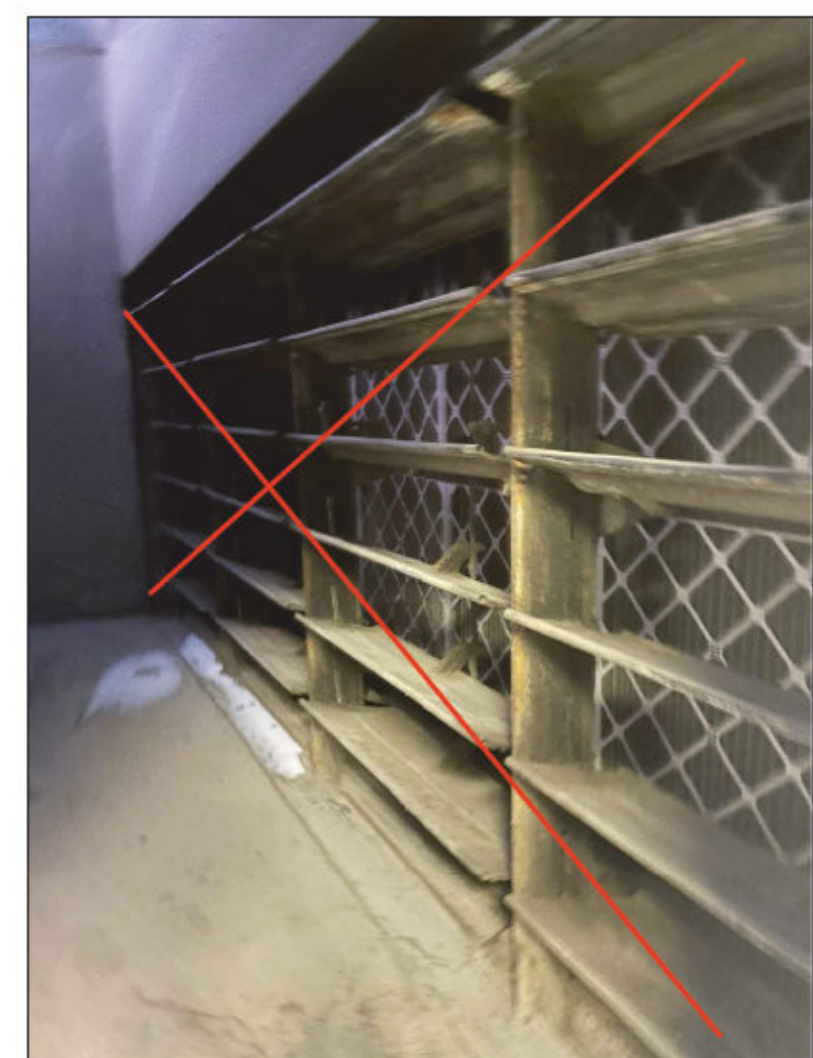
EXISTING DAMPER TO BE DEMOLISHED
