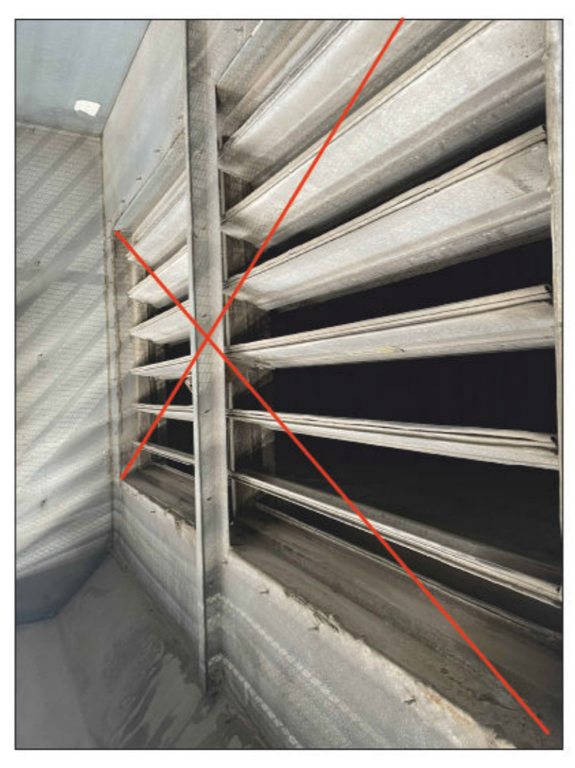
EXISTING DAMPER TO BE DEMOLISHED
